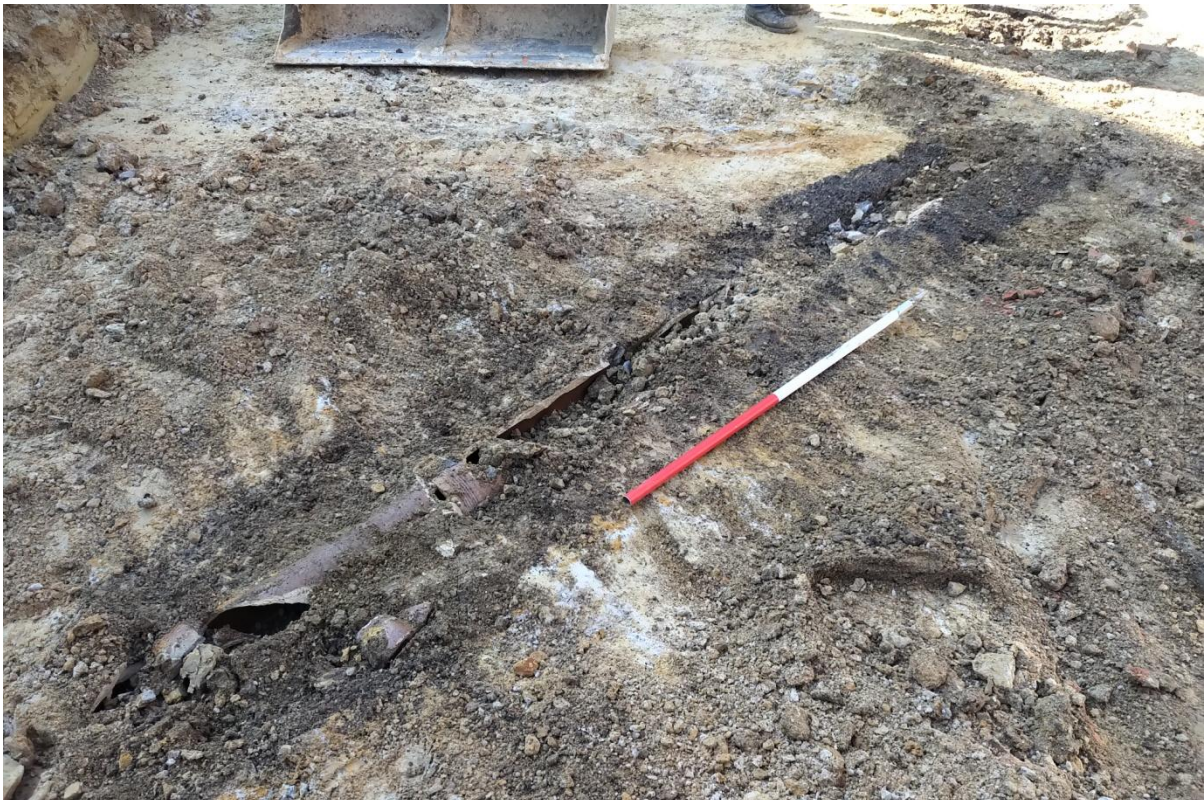
Plate 10: Provides more detailed overlook of exposed culvert. Looking south, one metre scale.
