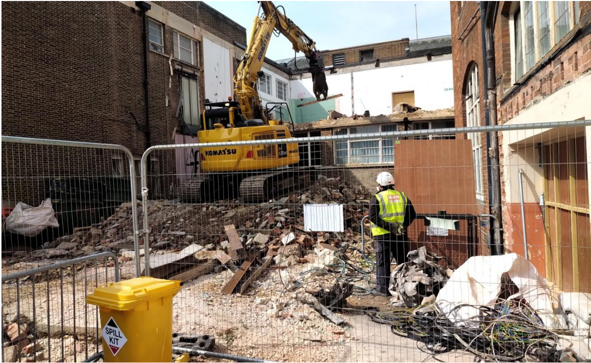
Plate 3: Showing on-going demolition of Lending Library. Looking west.
