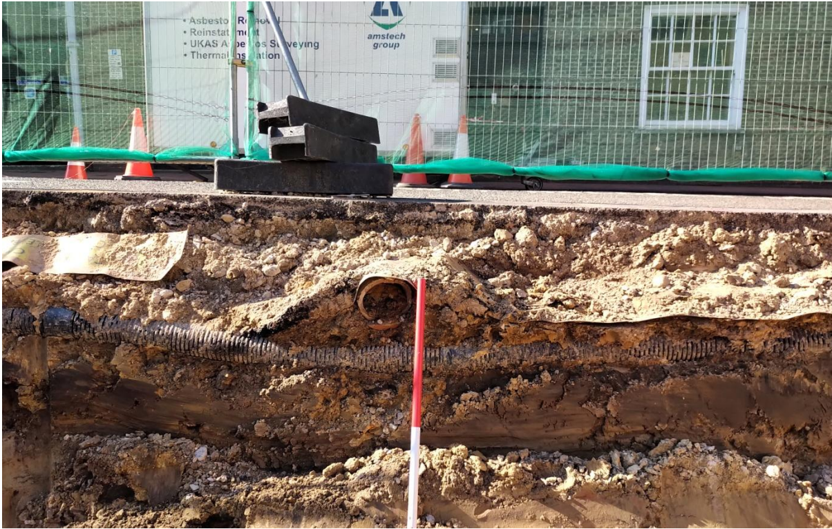
Plate 11: Culvert in southern section. Looking south with one metre scale.
